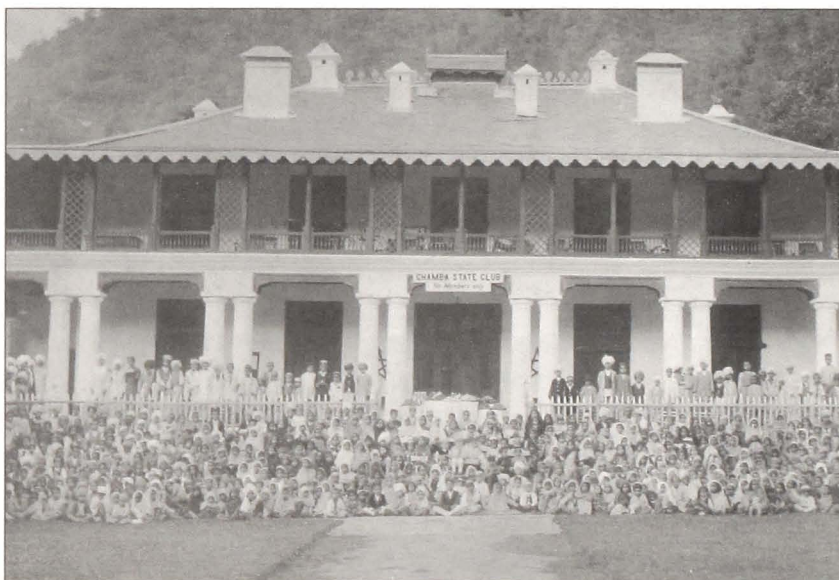
Building of the State Club, Chamba Photo courtesy: Manoj Kumar Vaid
