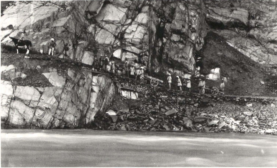
Engineer constructing the Hydro-electric Power House in Chamba Photo courtesy: Shri Pankaj Chowla
